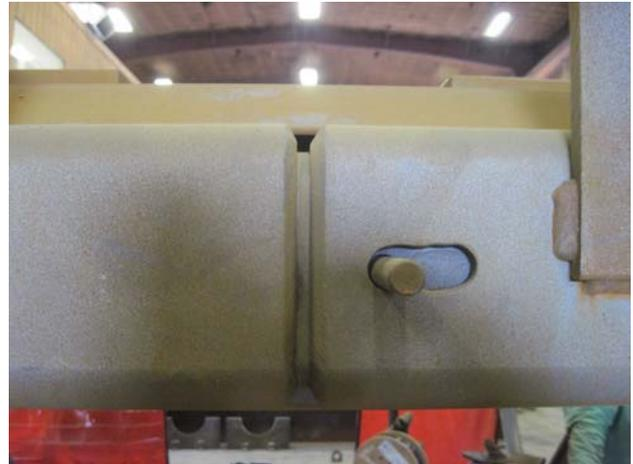
Figure 13: Splice detail, closed
