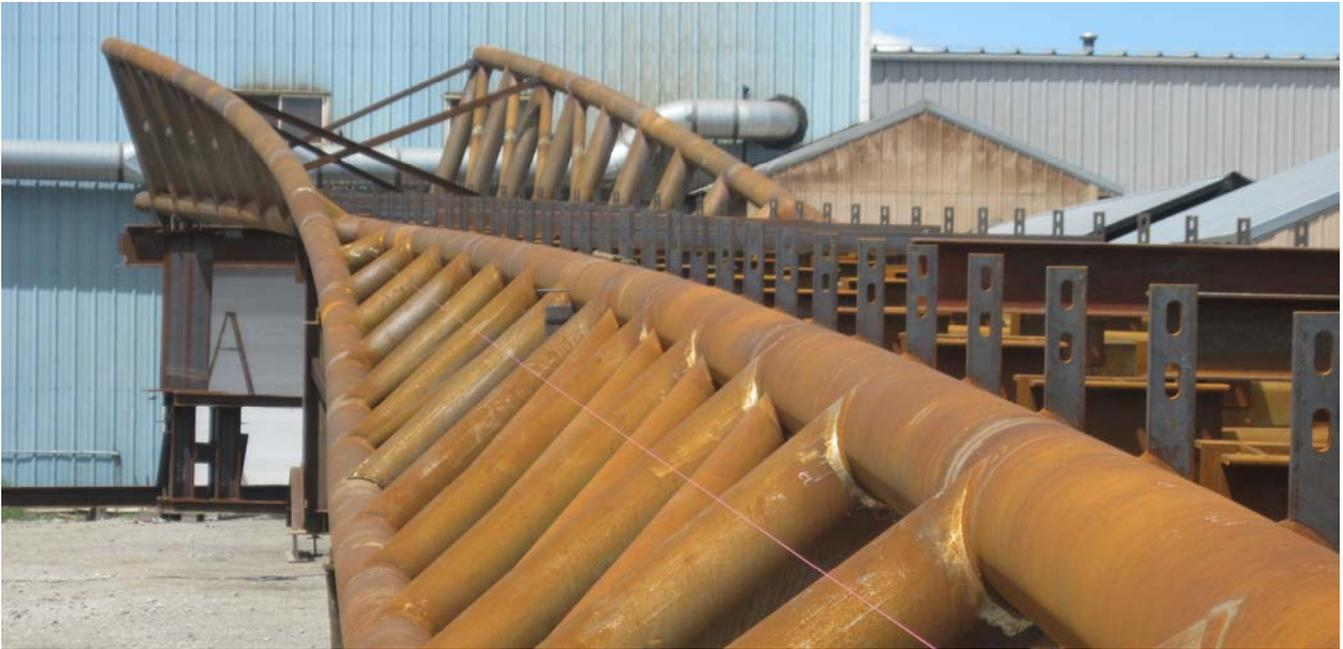
Figure 11: Partial pre-assembly in fabricator's yard
